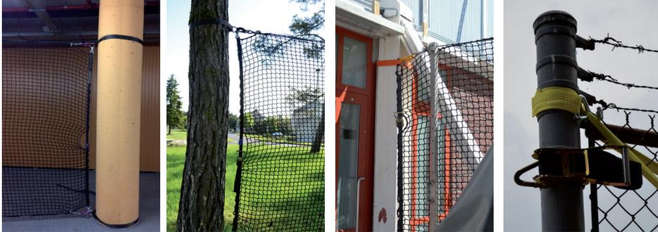
Prepare the lower anchor point by placing the ratchet strap around the object and make sure the fastening loop points towards the corresponding lower anchor point on the other side. Insert the strap end through the ratchet and tension. Arrange the upper anchor point by performing the same procedure as for the lower anchor point
