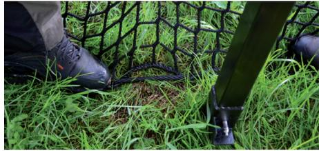
3. Tighten the upper wire pulley further to facilitate mounting of the support posts in the lower wire and prevent the support posts from swaying.
